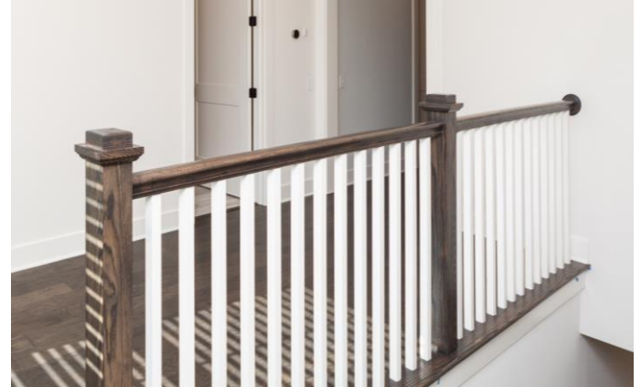
Arts & Crafts Stair Balusters
