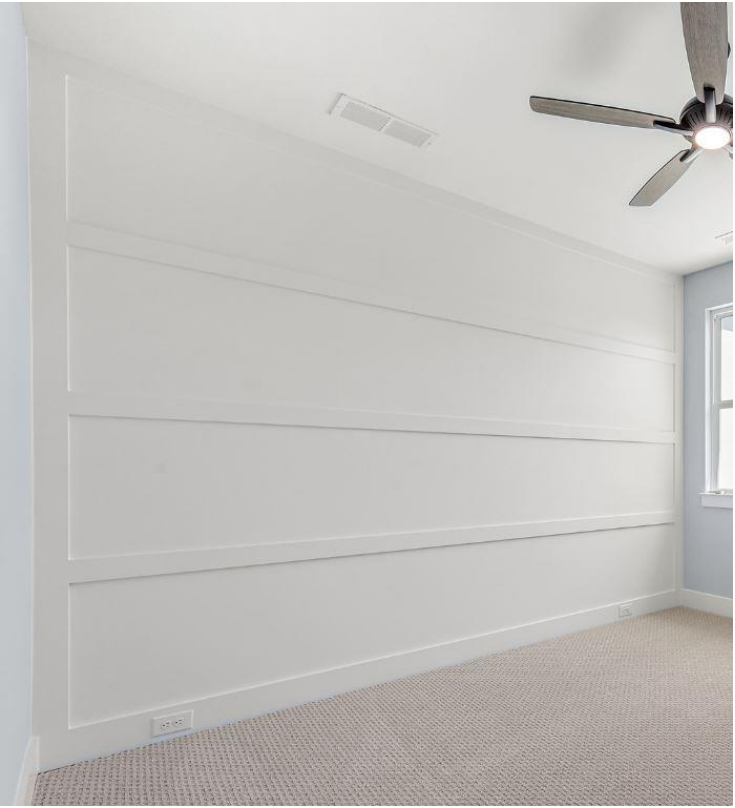
HORIZONTAL BATTEN STRIPS
